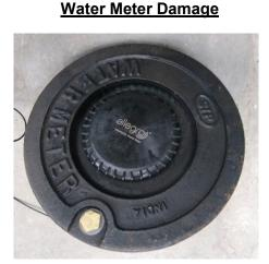
Our Water Department has started to upgrade our water meters to a new Master Meter Allegro meter. Some of you may have noticed a different-looking lid on your meter pit. It has a round black antenna in the middle of it. The antenna is connected to the water meter with a cable to boost the radio signal with the read from the meter. Removing the lid may <u>damage</u> the expensive electronics of the meter. The cost of repairing any damage caused <u>may be at the</u> <u>customer's expense.</u>
